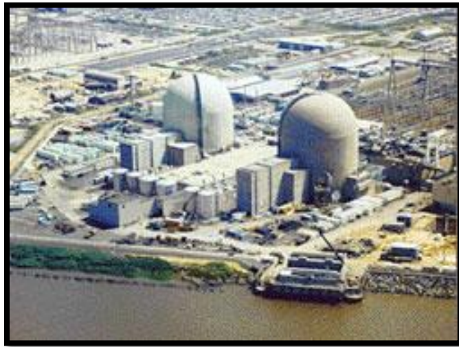
Figure 5. Salem Nuclear Power Plant Source: NRC
