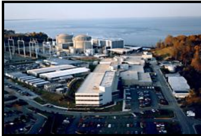
Figure 3: Calvert Cliffs Nuclear Power Plant Source: NRC
