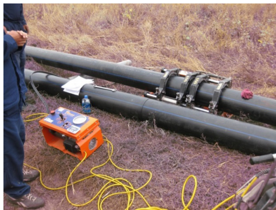
Workers use heat fusion to join replacement pipe sections. (Photo by OIG, September 2013.)
