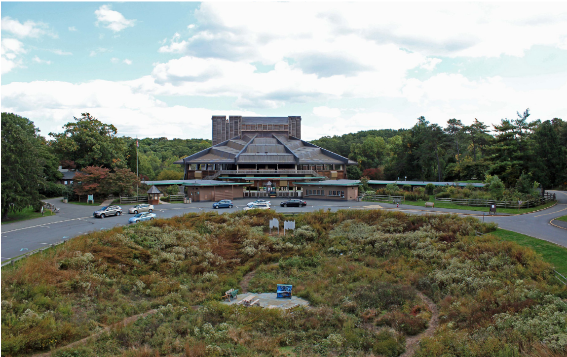
Aerial view of the Filene Center at Wolf Trap National Park for the Performing Arts.
