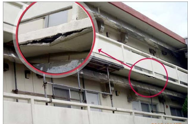
**Significantly deteriorated concrete building at Camp Futenma, Japan.**
