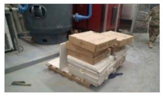
Storage of combustible material in mechanical room Source: DoD OIG.
