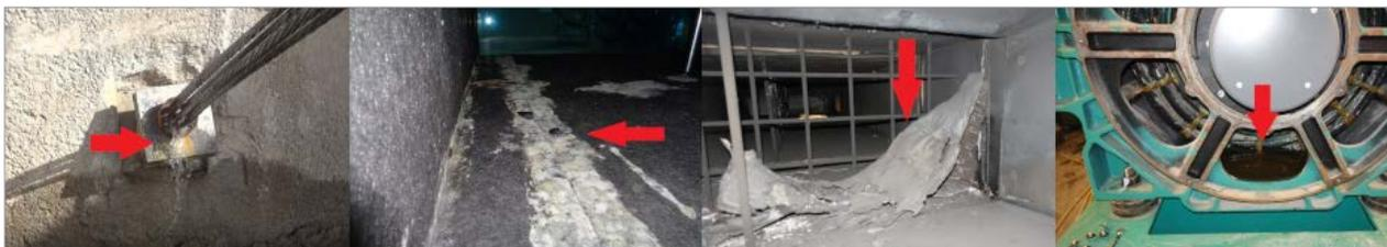
Photos are of water damage that resulted from the PERS wall not sealing properly in the USSTRATCOM facility in Omaha
