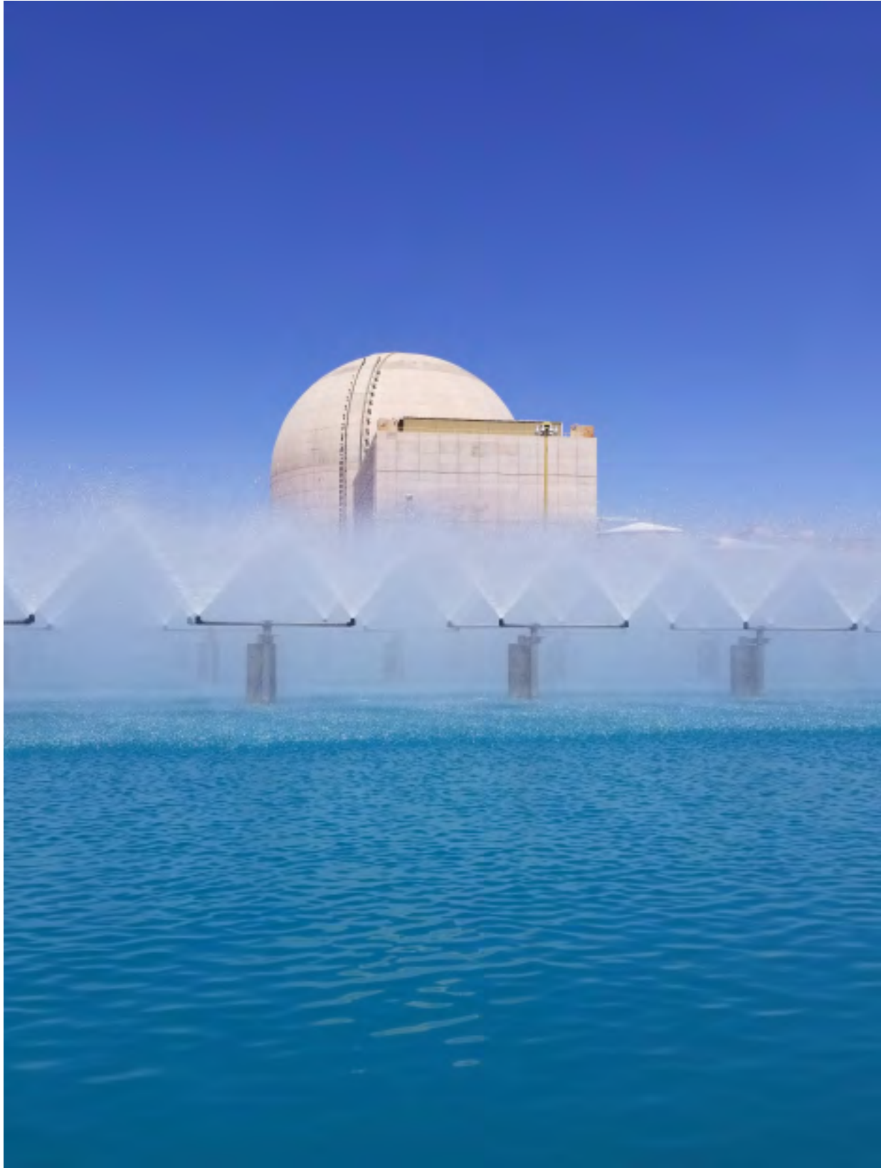
A spray pond at the Palo Verde Generating Station in the middle of the Arizona desert allows the plant to efficiently disperse heat from water used to cool some plant components.
