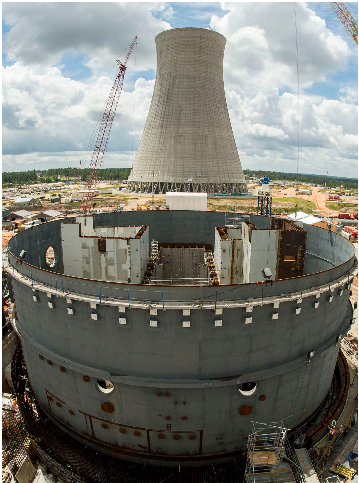
Vogtle Unit 3 nuclear island containment with cooling tower in background. Photo courtesy of Georgia Power
