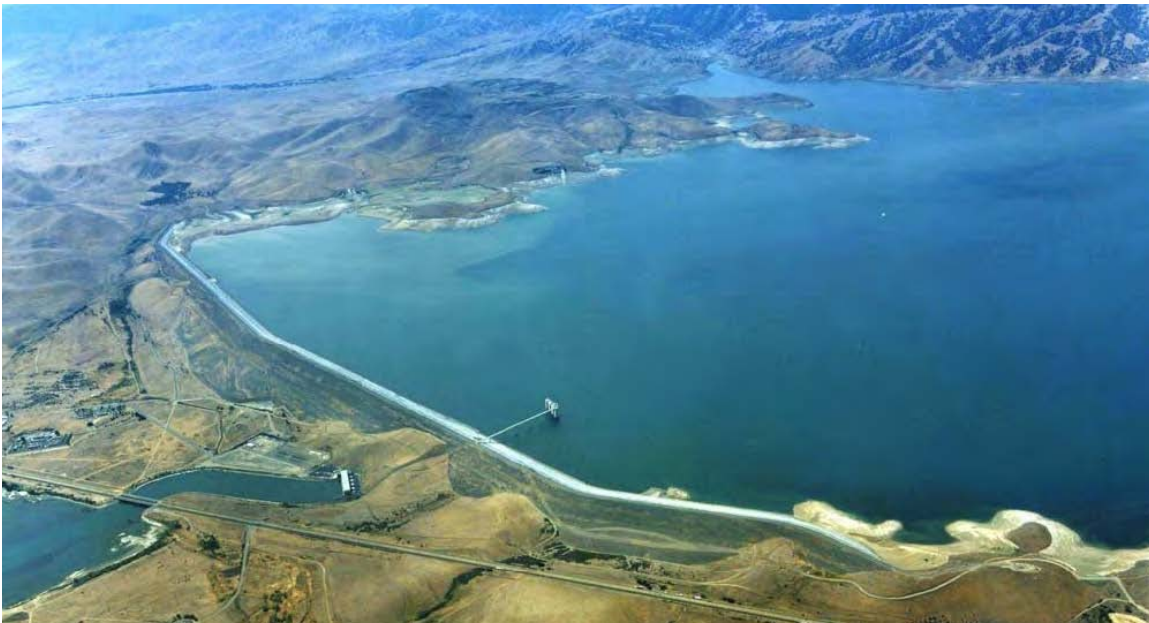
Aerial view of the San Luis Reservoir in Merced County, CA.
