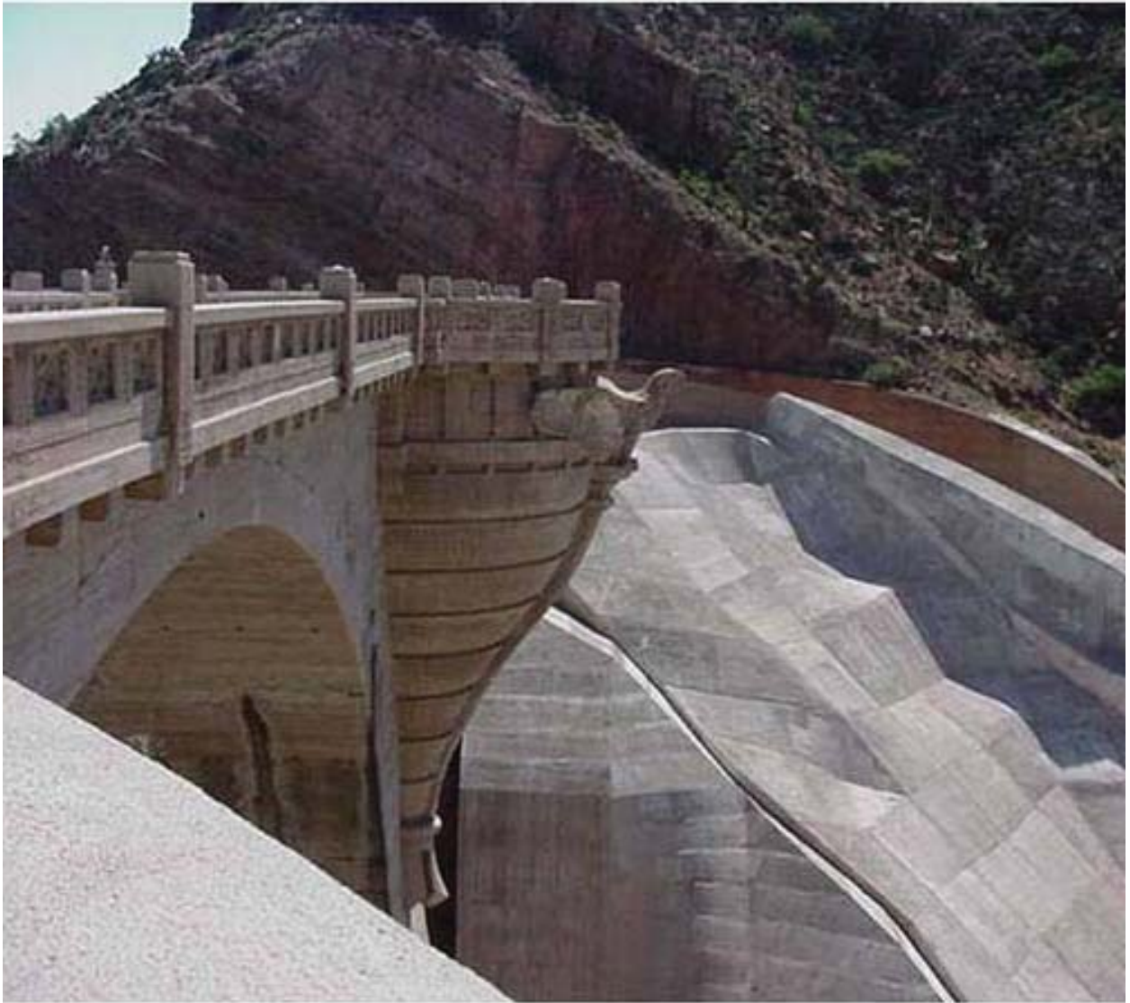
Coolidge Dam, San Carlos Irrigation Project, BIA
