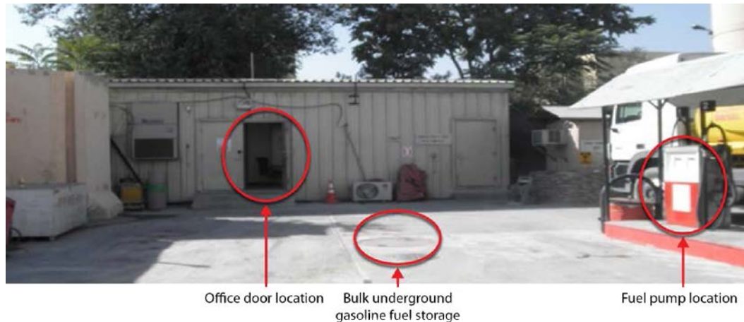
Figure 1: Fueling Station Office at Embassy Kabul
