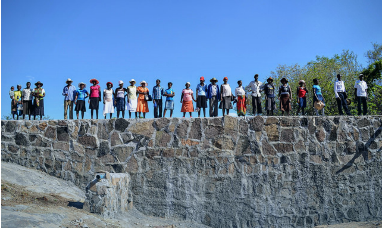
Community members in the Gwanda District of Zimbabwe stand on the Mbuyane dam, which they built as part of a USAID-funded cash-for-assets activity. Photo: USAID/Zimbabwe (Oct. 25, 2015)
