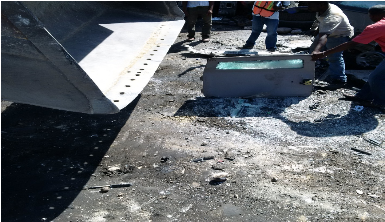
Figure 7. Contractor personnel, with no personal protective equipment, holding an armored door while the front-end loader attempts to smash it.
