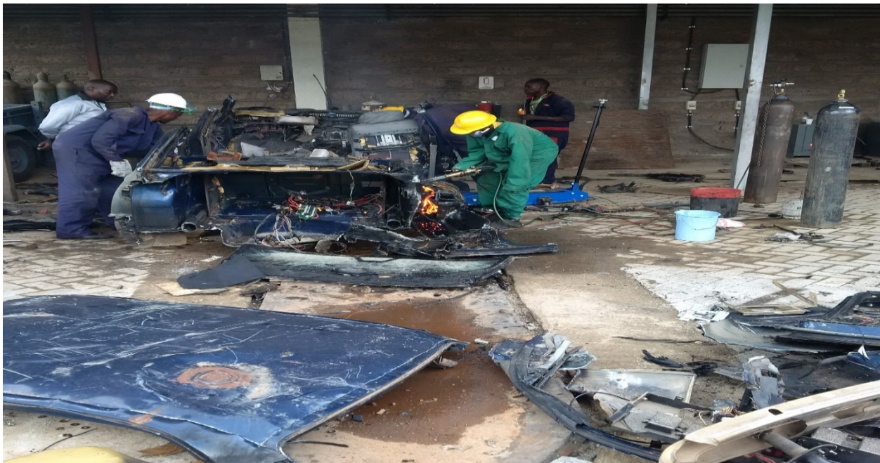
Figure 2. Contracted workers using a blow torch in an enclosed area; two contractors supervising the disposal lack the required personal protective equipment.
