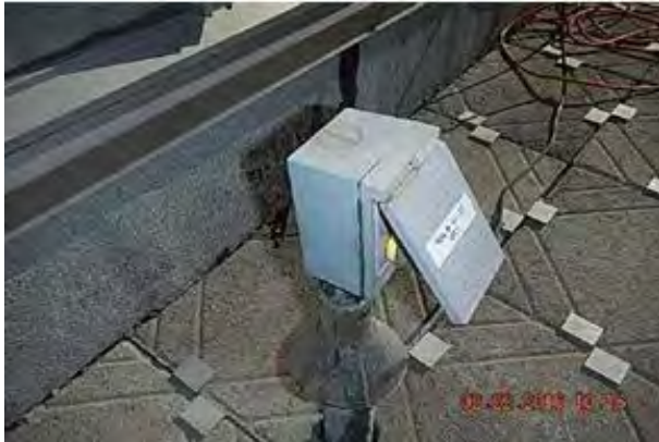
Figure 5: Unattended, Plugged-in Device Without a Waterproof Enclosure in SDA-1.
