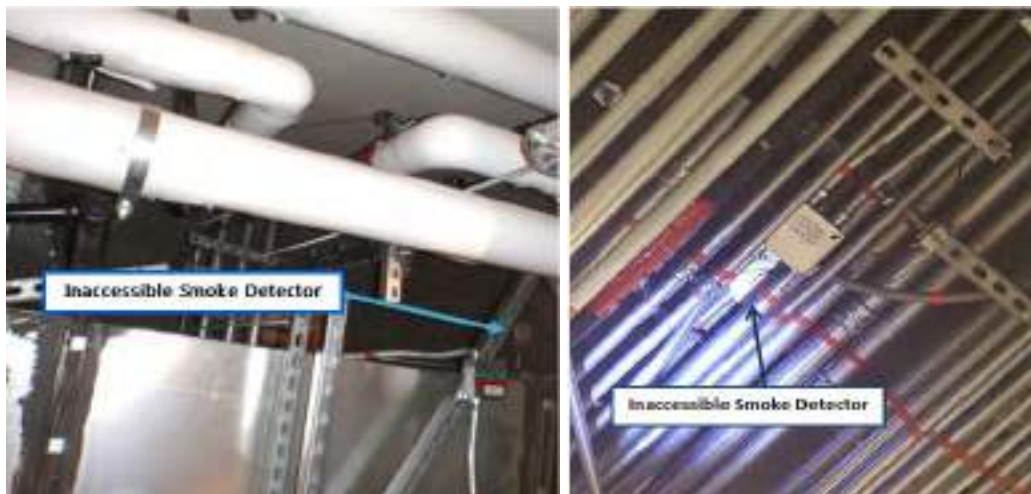
Figure 6: Smoke Detectors in the NOX Inaccessible for Testing and Maintenance.
