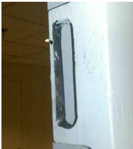
Figure 3: Example of a Ground-Down Strike Plate to a Security Door in SDA-1.
