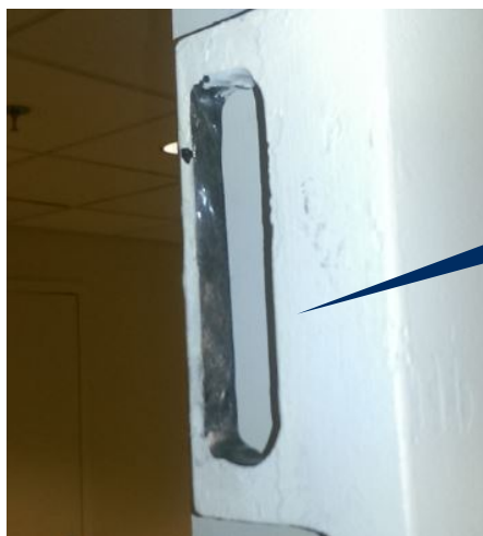
Figure 2: Example of ground-down strike plate to a security door in SDA-1
