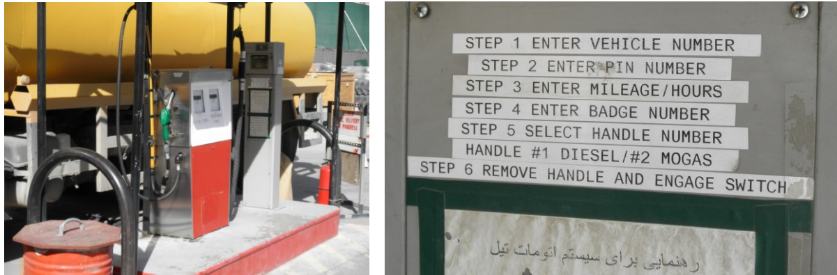
Figure 2: Kabul Embassy's Fueling Station and directions for using the fuel system.
