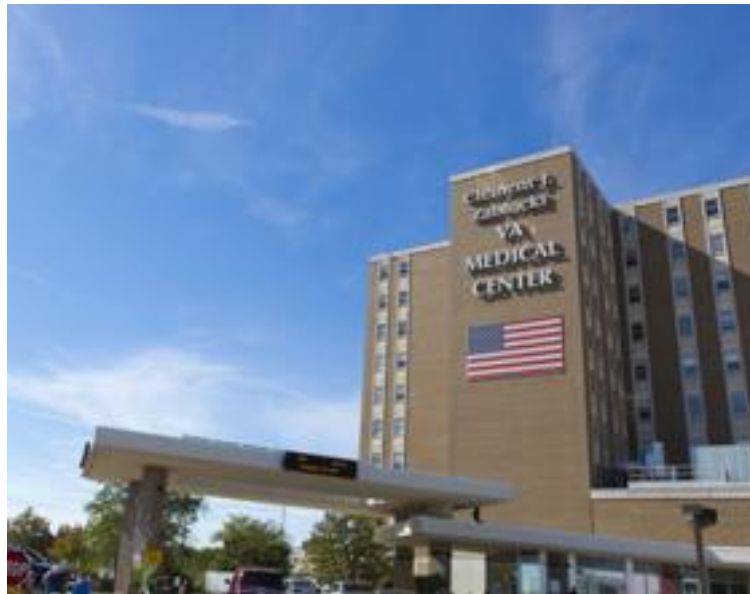
Figure 1. Clement J. Zablocki VA Medical Center in Milwaukee, Wisconsin (Source: https://vaww.va.gov/directory/guide/ , accessed on January 28, 2020)
