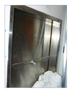
Figure 13. A photo of an unlocked dumbwaiter in a telecommunications room.
