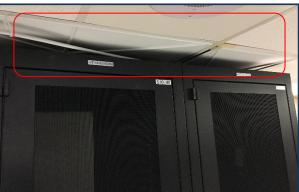
Figure 8. (Left) Picture of the proximity of the sprinkler heads to the server racks in the data center room, taken during the audit team's inspection.
