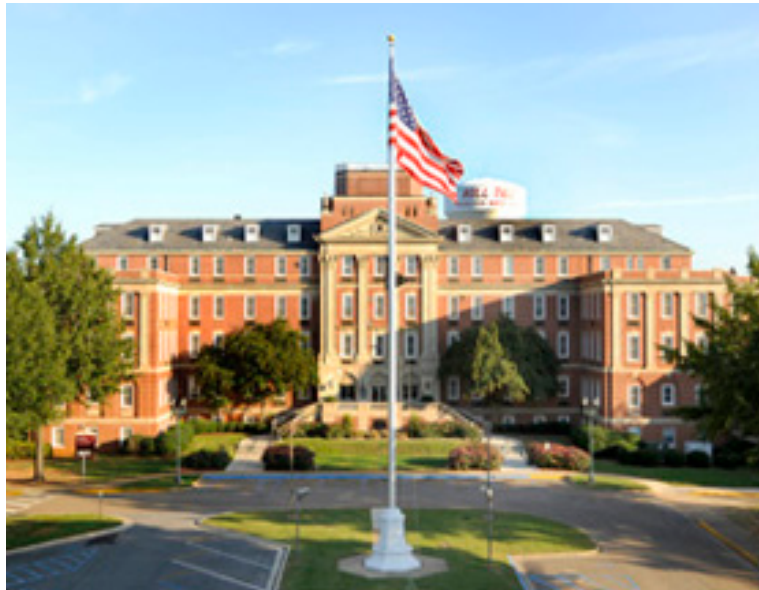
Figure 1. Tuscaloosa VA Medical Center, Tuscaloosa, AL (Source: https://vaww.va.gov/directory/guide/ , accessed on May 22, 2019)
