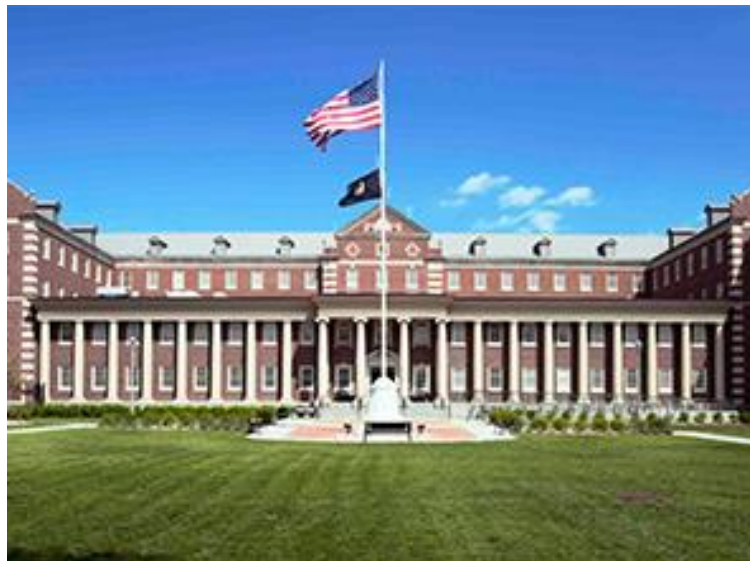
Figure 1. Fargo VA Health Care System, North Dakota (Source: https://vaww.va.gov/directory/guide/ , accessed on July 22, 2019)
