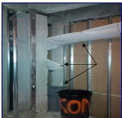
Figure 3. SICU Project: Construction Area Open to Weather, Water Diversion, and Collection
