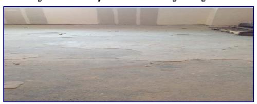
Figure 6. SICU Project: Uneven and Fragmenting Floor
