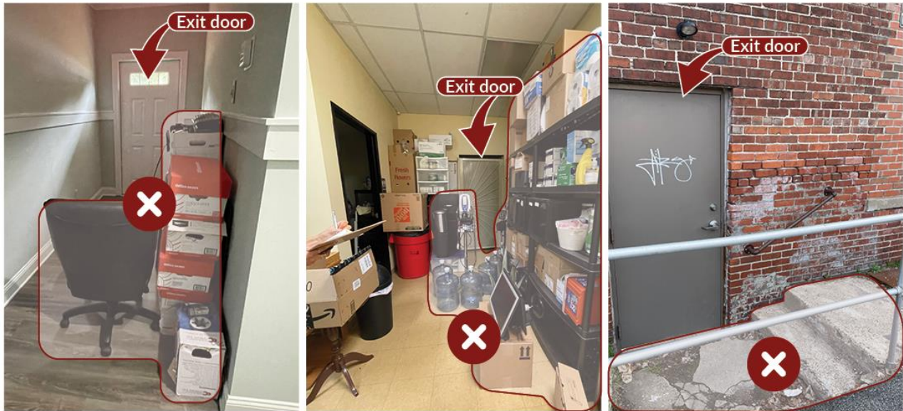
Figure 7. Exit route issues in contract exam facilities in South Carolina (left), Arizona (center), and New York (right).
