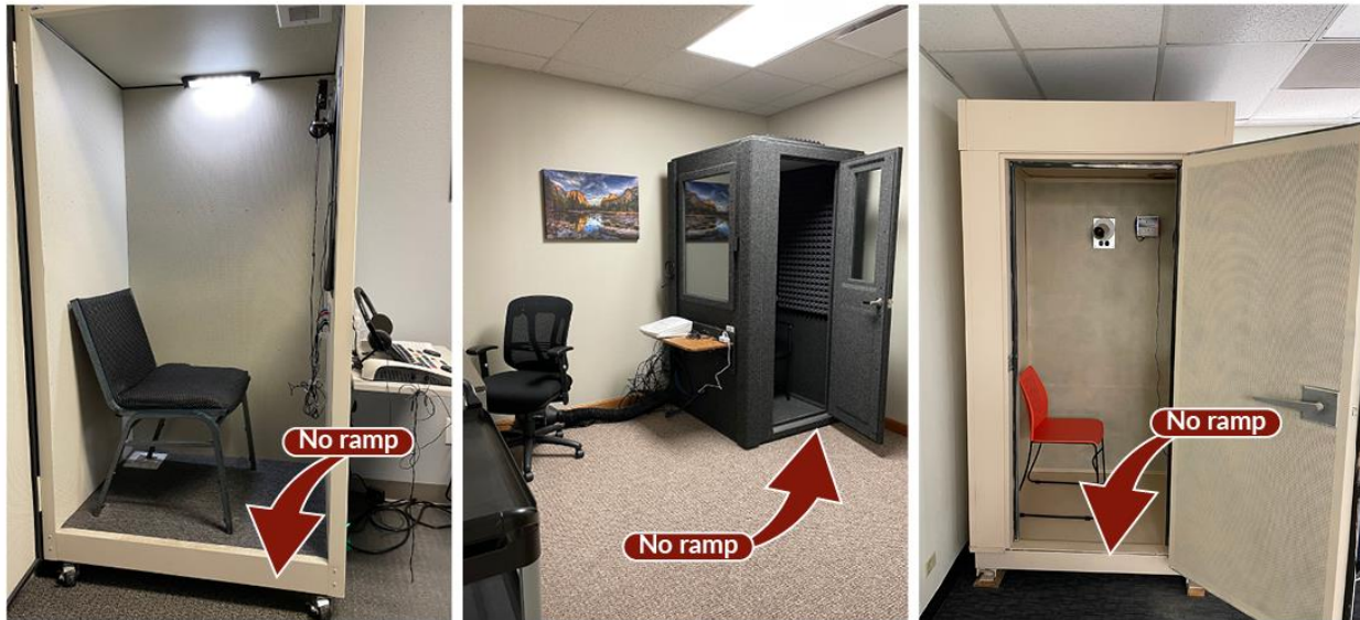
Figure 6. Audio booth accessibility deficiencies at contract exam facilities in Texas (left), Wisconsin (center), and Missouri (right).
