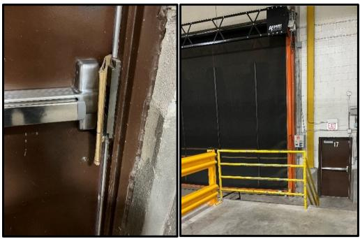
*Figure 9.* Blocked door-locking mechanism in the Hines warehouse. Source: VA OIG, July 13, 2022.
