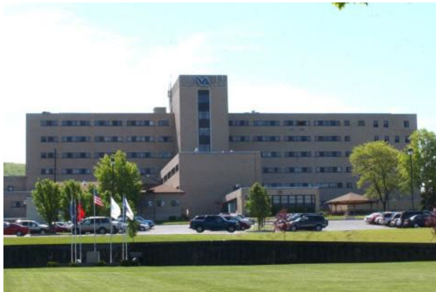
Figure 1. James E. Van Zandt VA Medical Center in Altoona, Pennsylvania. Source: https://www.va.gov/altoona-health-care/locations (accessed January 31, 2023).
