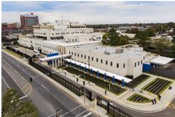
Figure 1. Memphis VA Medical Center in Tennessee.
