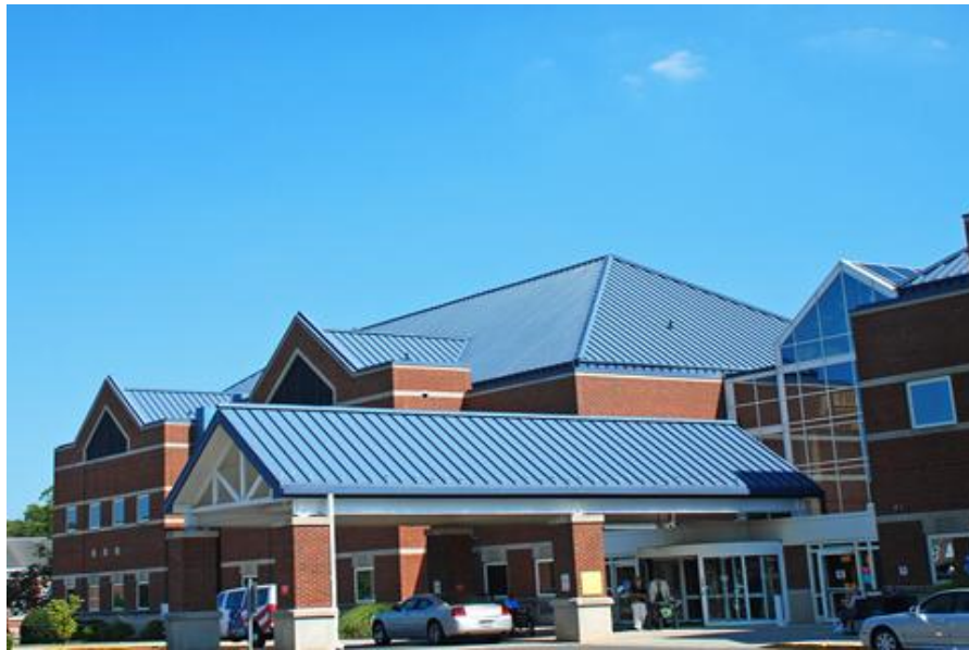
Figure 1. Northport VA Medical Center in New York.
