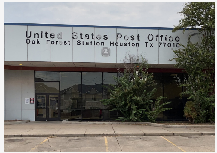
Figure 7. Missing Letters in Signage
