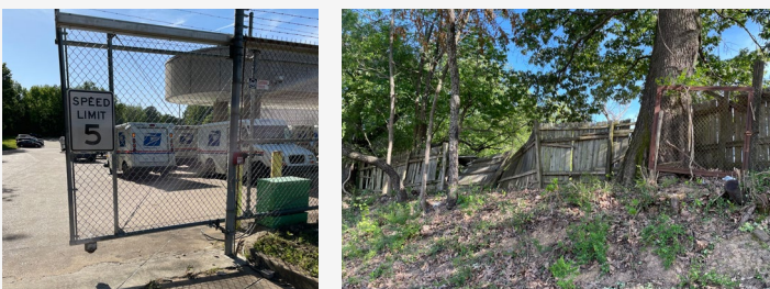
Figure 3. Unsecured Gate and Perimeter Fence
