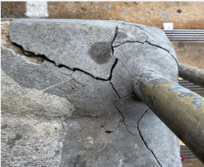
Figure 7. Cracked Concrete
