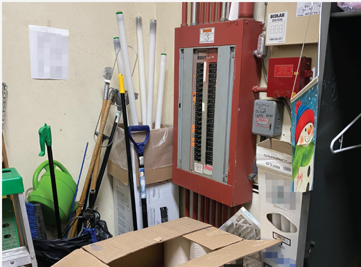
Figure 4. Blocked Electrical Panel
