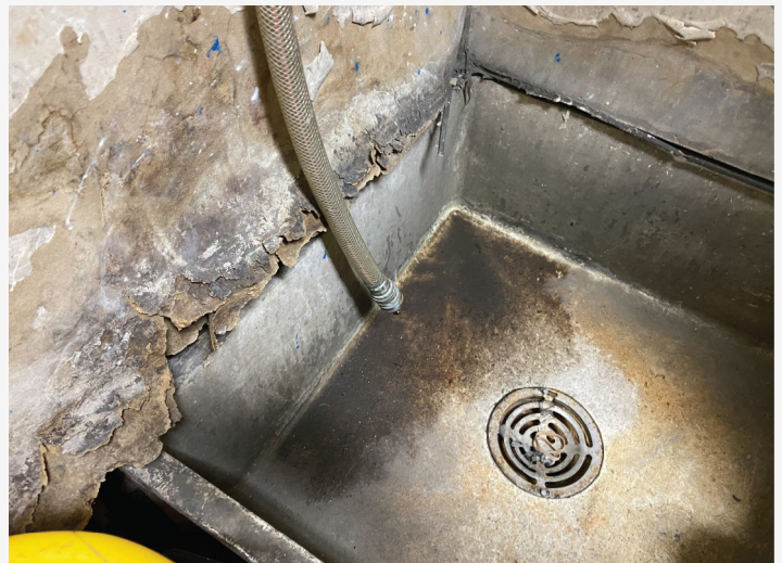
Figure 5. Damaged Walls at the Custodian Sink
