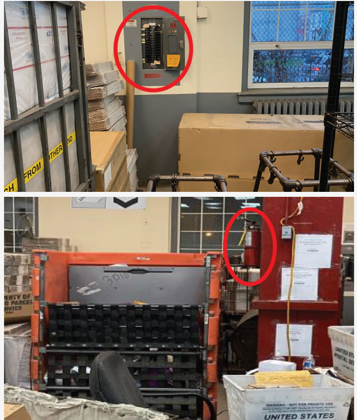
Figure 4. Blocked Electrical Panel and Fire Extinguisher
