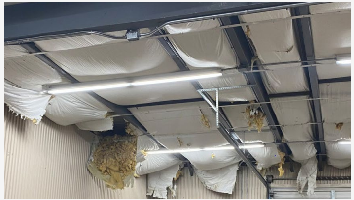
Figure 5. Damaged Ceiling
