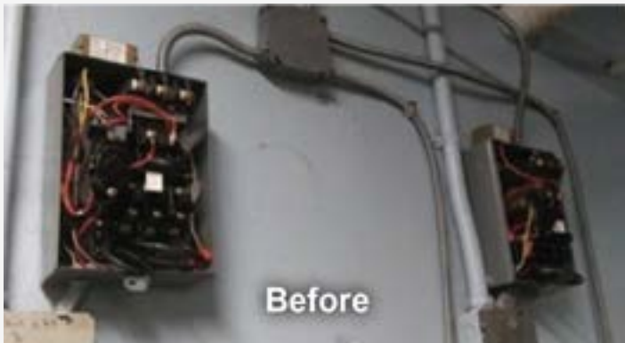
Figure 5. Exposed Wiring
