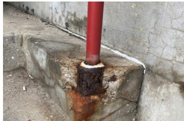
Figure 8. Rusted Handrail
