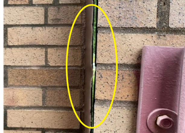
Figure 7. Inspection Gate Pulling Wall Apart
