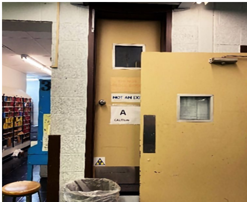
Figure 14. Blocked Inspection Service Door
