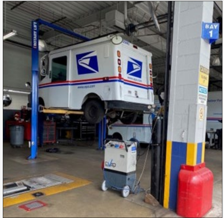
Figure 2. Potentially Inadequate Spacing Between Ceiling and Lift Height
