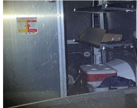
Auburn Park Station
