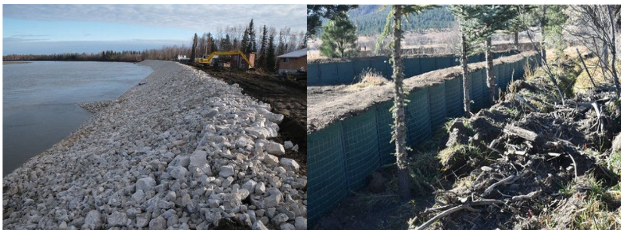
Figure 3: (Left) Emergency response (streambank stabilization). Photo from NRCS Alaska's Flickr account. (Right) Barriers used for wildfire recovery. Photo from NRCS New Mexico's Flickr account. The photos do not depict any particular audit, inspection, or investigation.
