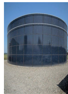
Waste Storage Facilities
