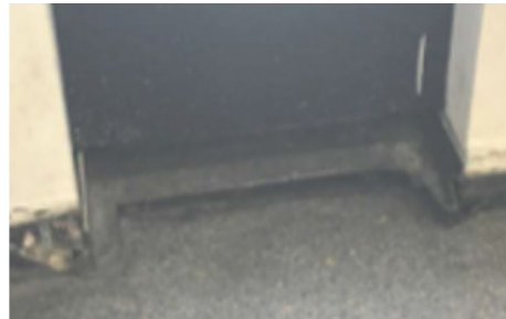
Crack Between Baseboard and Floor.
