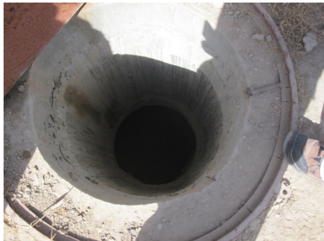
Photo 4 - Access Point to Septic Tank
