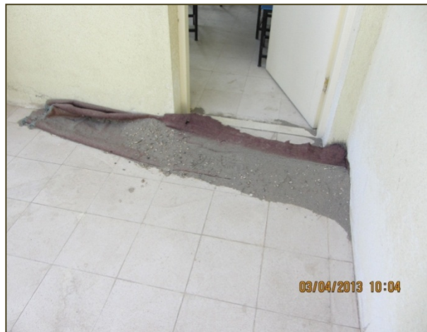
Photo 3 - Improvised Dam on Sloping Roof Terrace
