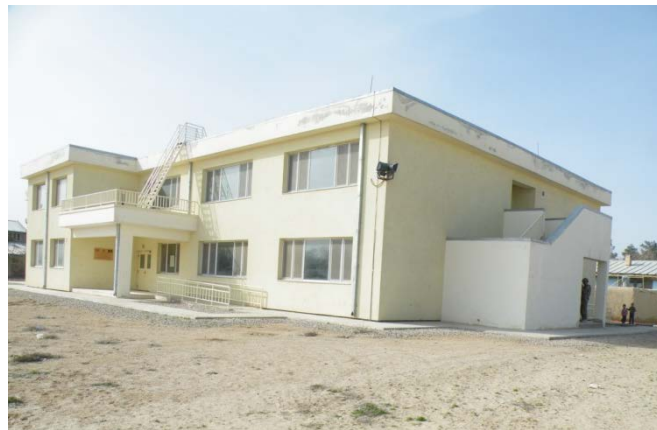
Photo 1 - Balkh Education Facility
