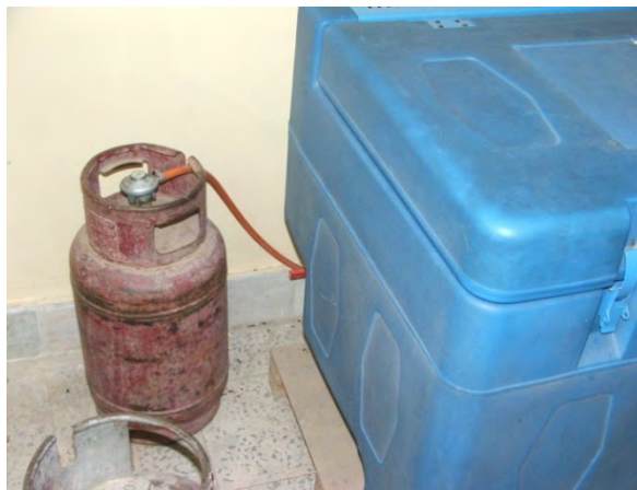
Photo 4 - Propane Supply for Refrigerator
