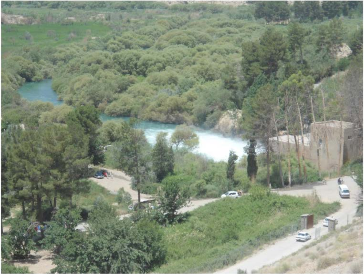
The photograph above of the Kajaki Dam, which was rebuilt under CLIN 5, was taken by Horwath MAK, Crowe Horwath LLP's Afghanistan affiliate, during in-country observation and inspection activities pertaining to the audit of BVSPC's Special Purpose Financial Statement.
