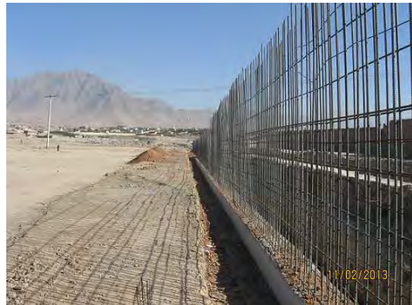
Photo 2 - Perimeter Wall Foundation and Reinforcing Steel
