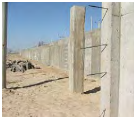
Photo 3 - Perimeter Wall and Column for Guard Tower
