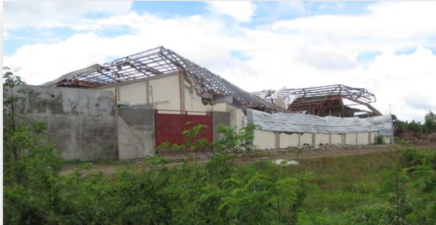
Figure 2. Warehouse Damaged by Typhoon Yolanda
