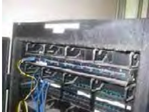
Figure 6- Dust covered Sensitive Equipment
