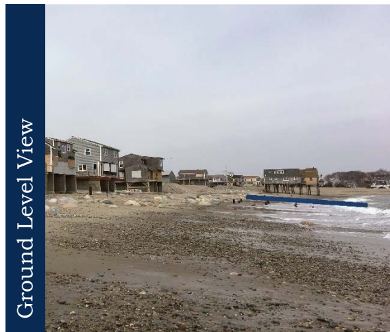
Ground level view of FEMA acquired and demolished SRL Property (see blue line) Source: OIG photo
