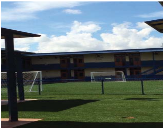
Figure 1. Recreation field at Karnes Source: Office of Inspector General (OIG)
