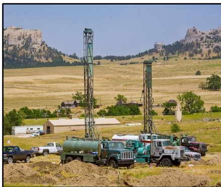
In-situ Uranium Recovery, Crow Butte, Nebraska (Source: Courtesy of Cameco Corp.)
