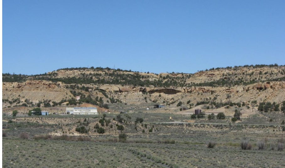
The Church Rock uranium mill tailings site in Gallup, NM Source: OIG, NRC
