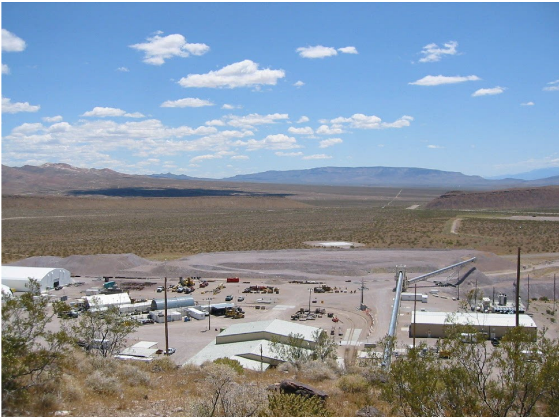
The excavation and development facilities at Yucca Mountain.
